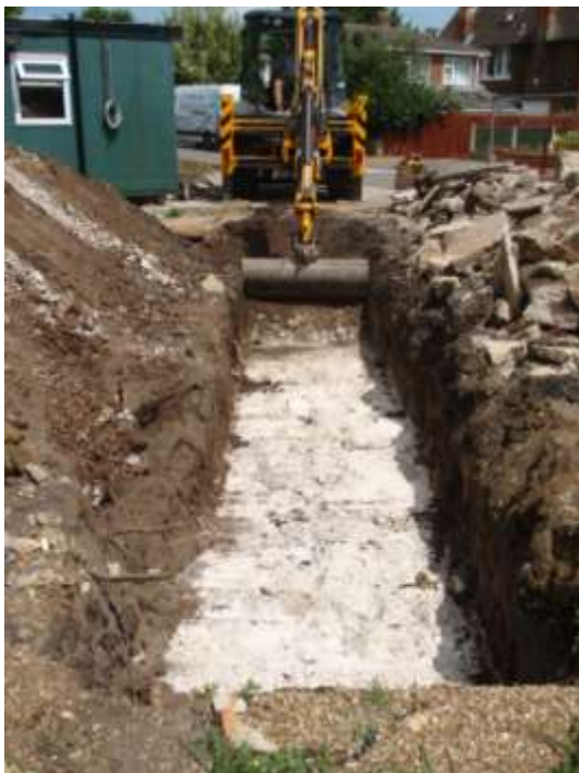
Plate 3. Trench 1 (looking NNE)
